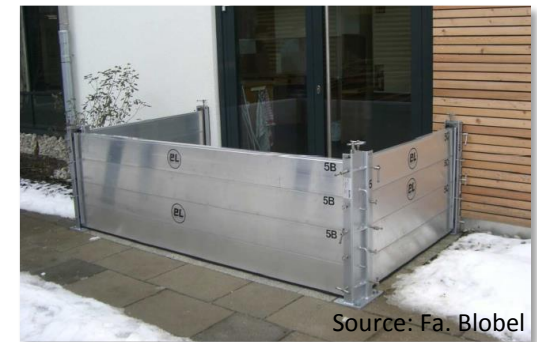
mobile flood barriers
