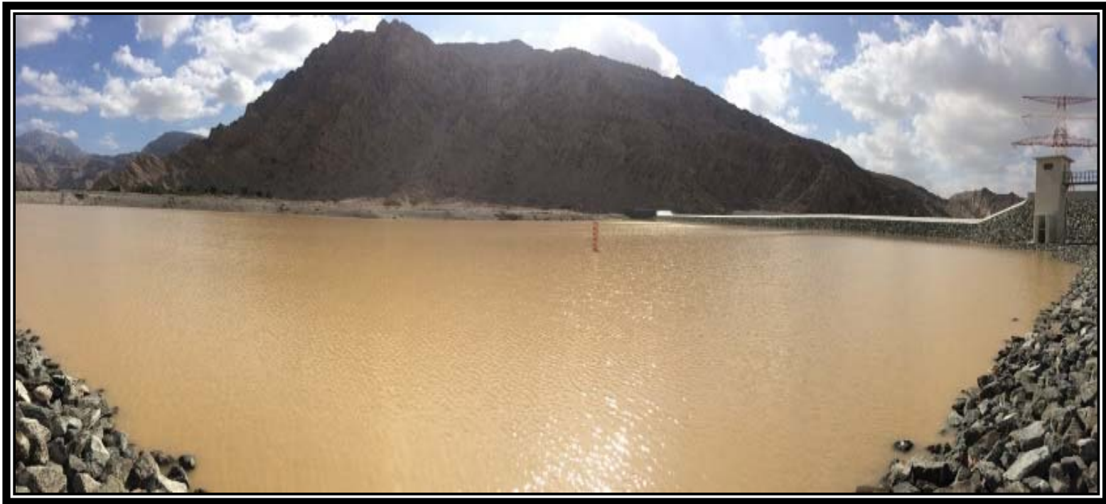
Dam reservoir conditions after stormy weather
