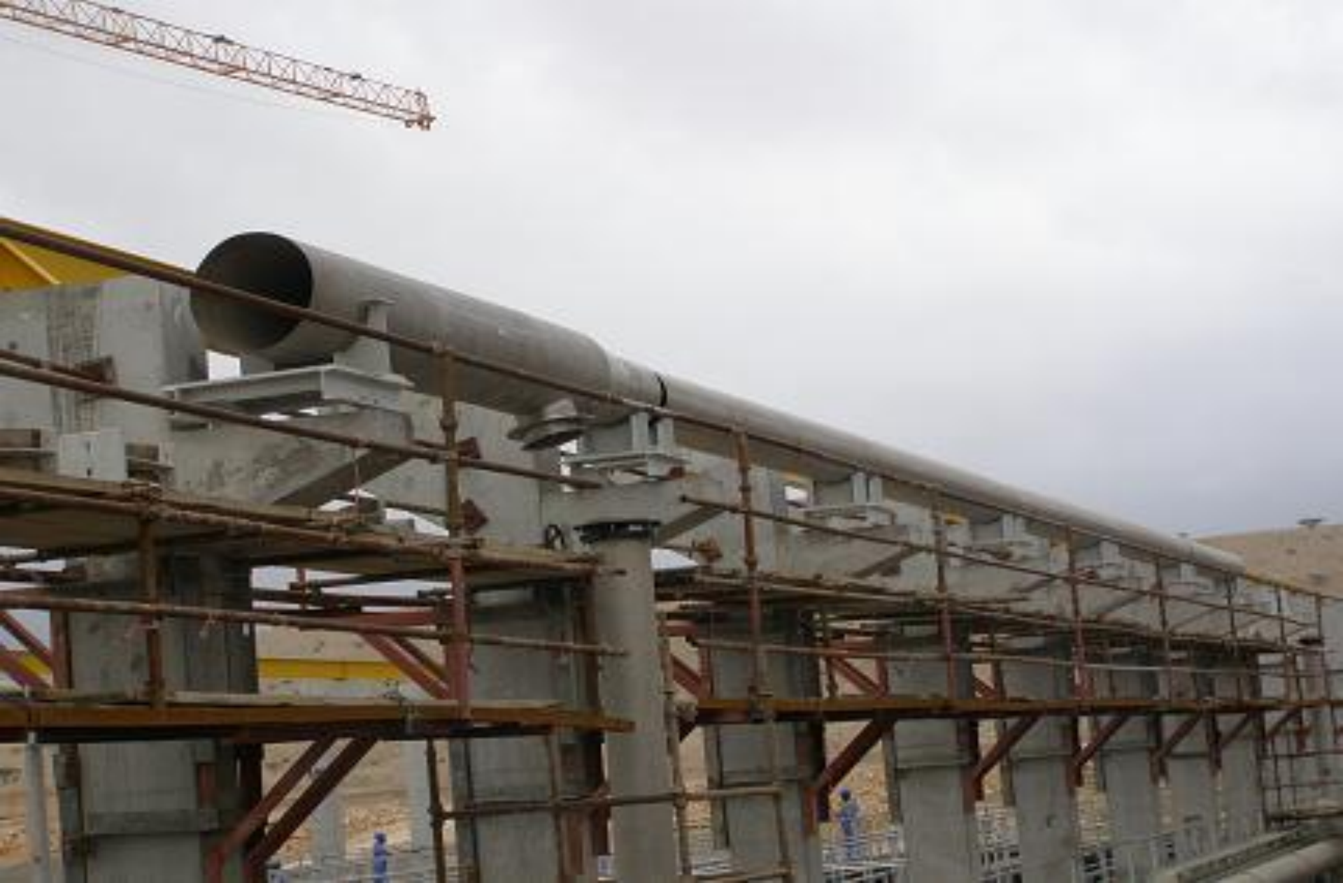
Installation of Air Headers above biological aeration tanks
