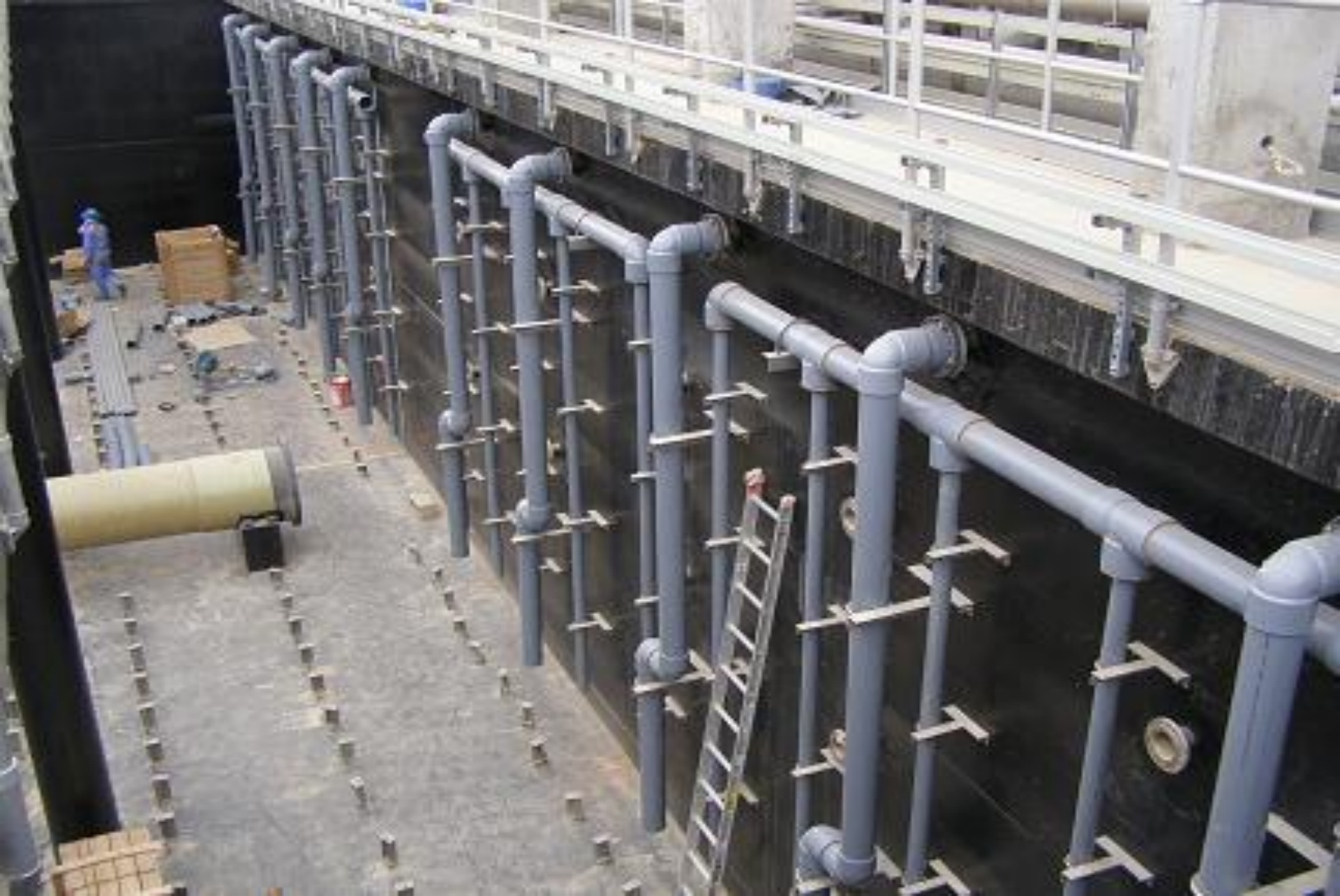
Installation of piping work in membrane Tank 7
