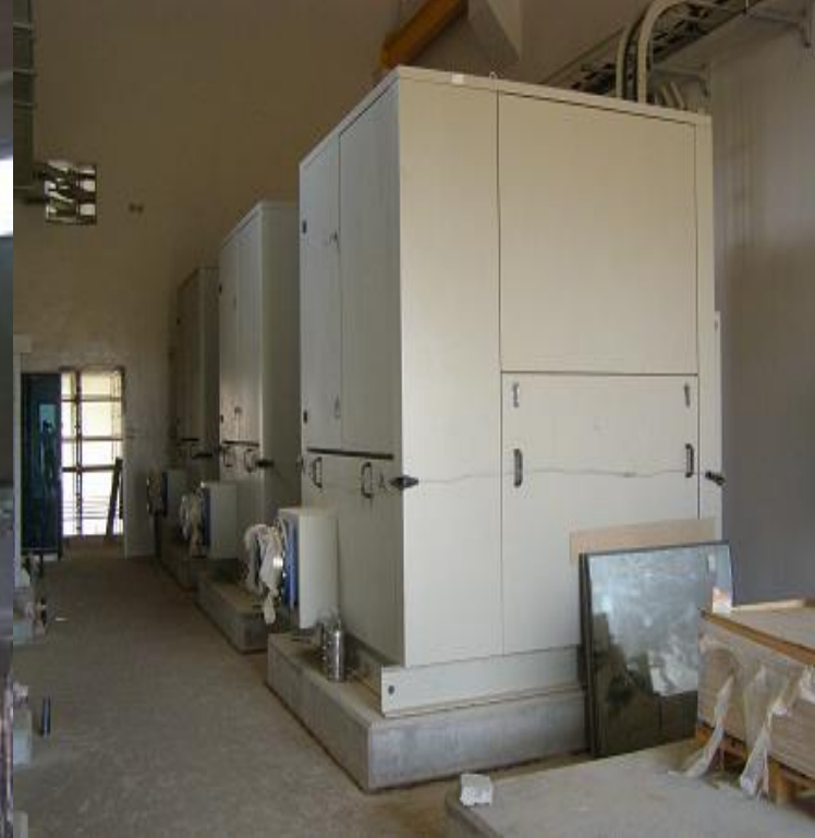
Installation of PD Blowers
