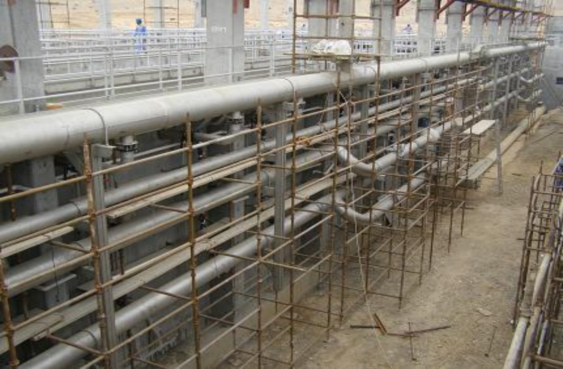
Air & Permeate Header Piping outside membrane Tanks 5
