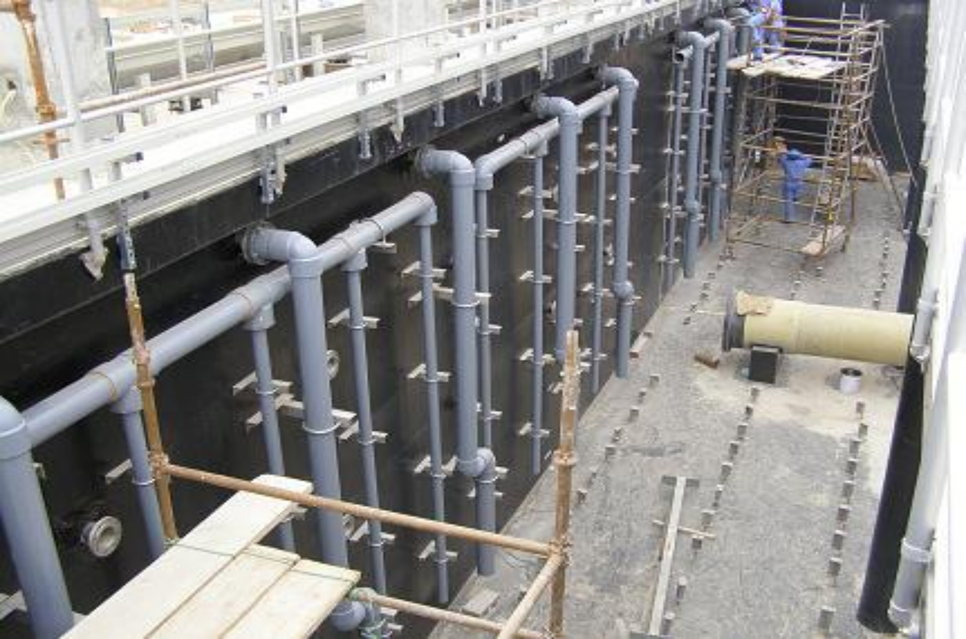
Installation of piping work in membrane Tank 8
