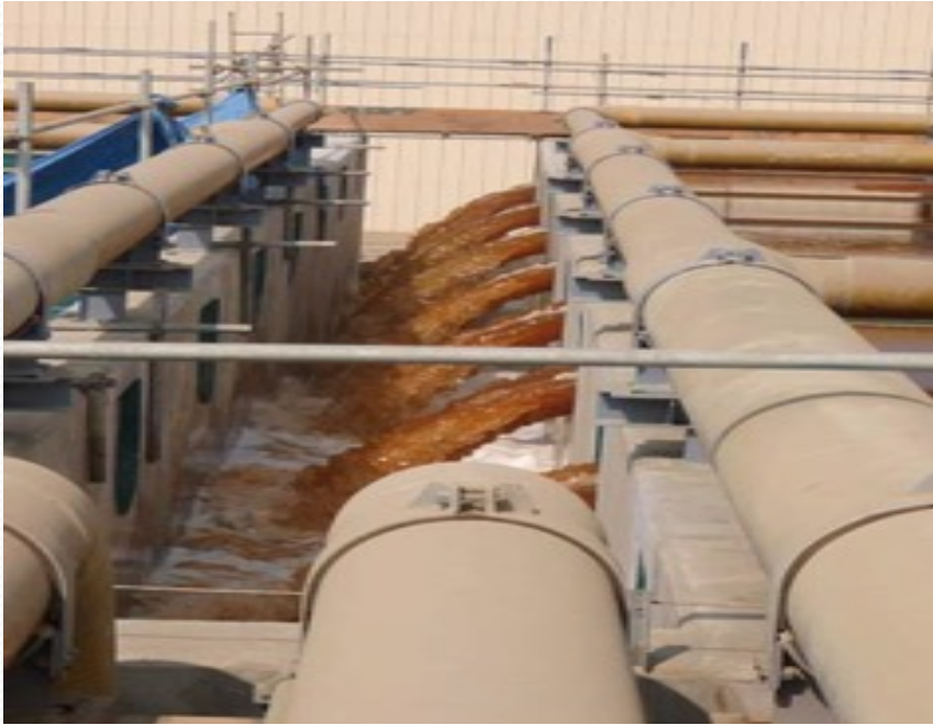
Figure 3. The issue with current air flotation process: the brown color of treated effluent, which is stained by the industrial coagulants ( ferric chloride ), and non-biodegradable sludge
