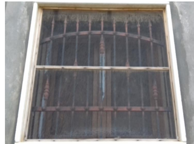
Figure 5. Window's protection from mosquitoes attack
