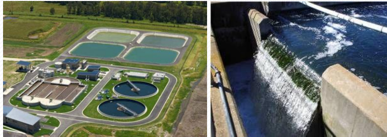
Sewage Treatment Plant (STP)
