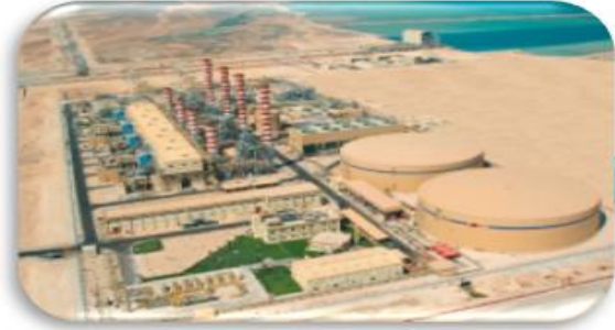
Water Desalination Plant
