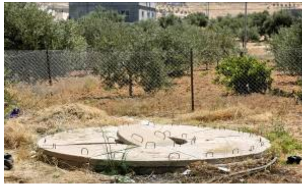
Figure 3. Concrete greywater treatment-circular design
