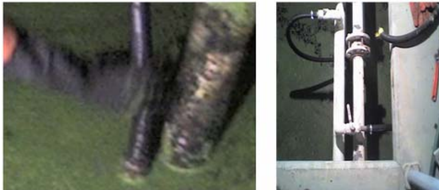
Figure 9: Insering New Hose at bottom end. Figure 10: New Hose clip Fixing
