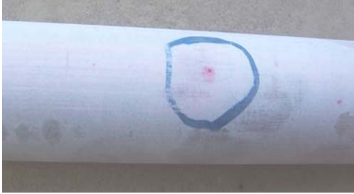
Figure 11. Closer view showing nucleation of pits after dye penetration test
