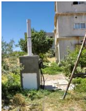
Figure 4. Concrete greywater treatment-rectangular design
