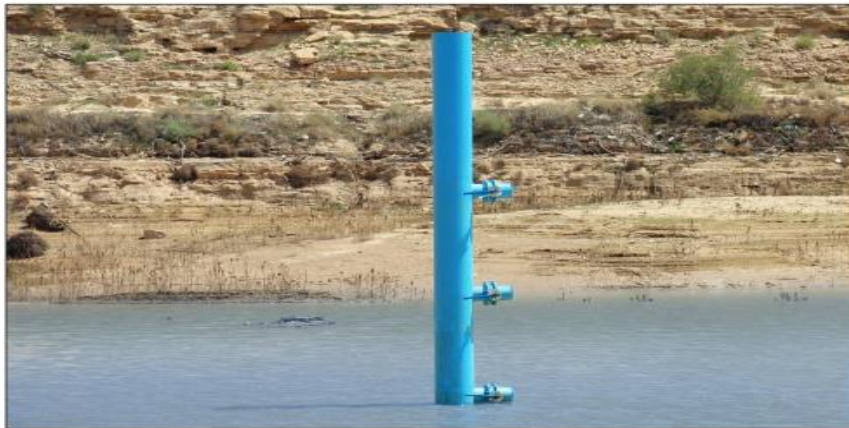
Ground water recharge in Al Ulb Dam (Ad Dariyah)
