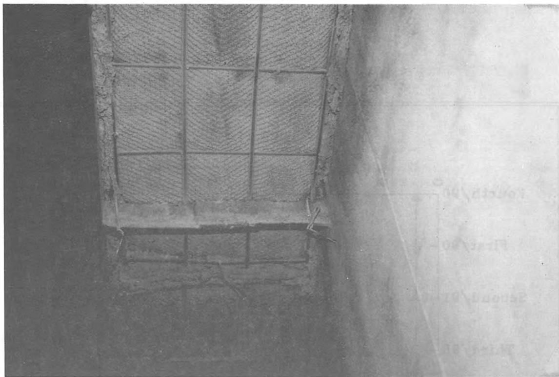
STAGE 1 - DEMISTERS COVERED WITH HARD SCALE
