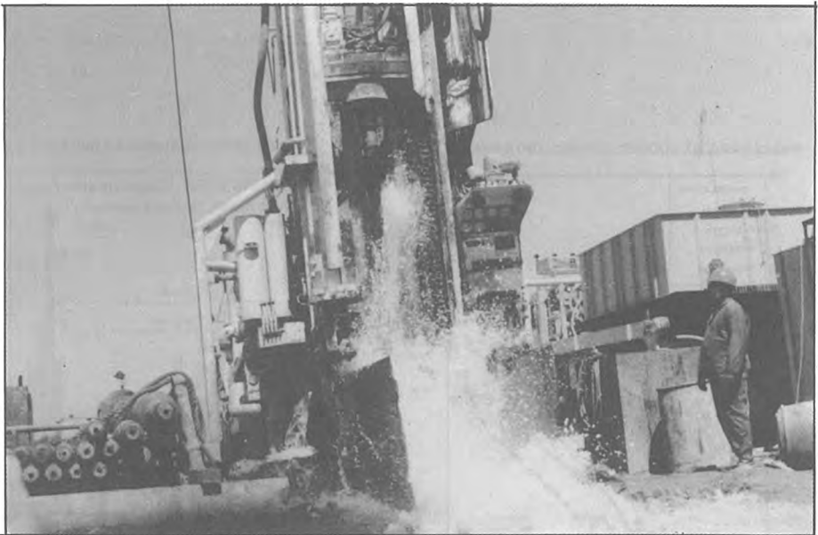
Figure 3. Air-foam rotary drilling rig, ND-86.
