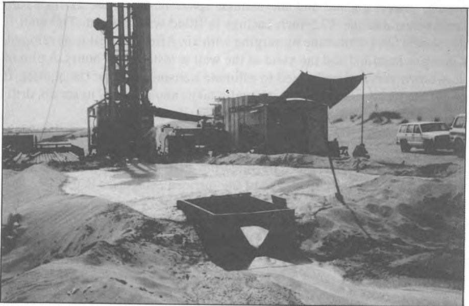
Figure 4. V-notch weir used to gage outflow from the borehole during drilling.
