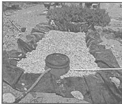
Figure 2: Confined Trench Greywater Treatment Unit
