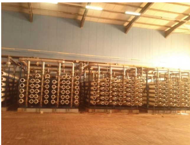
Fig. 1. Spiral wound membrane modules in the Tajoura desalination plant.
