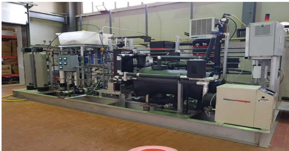
Fig. 4. Pilot scale FO-thermal test unit.
